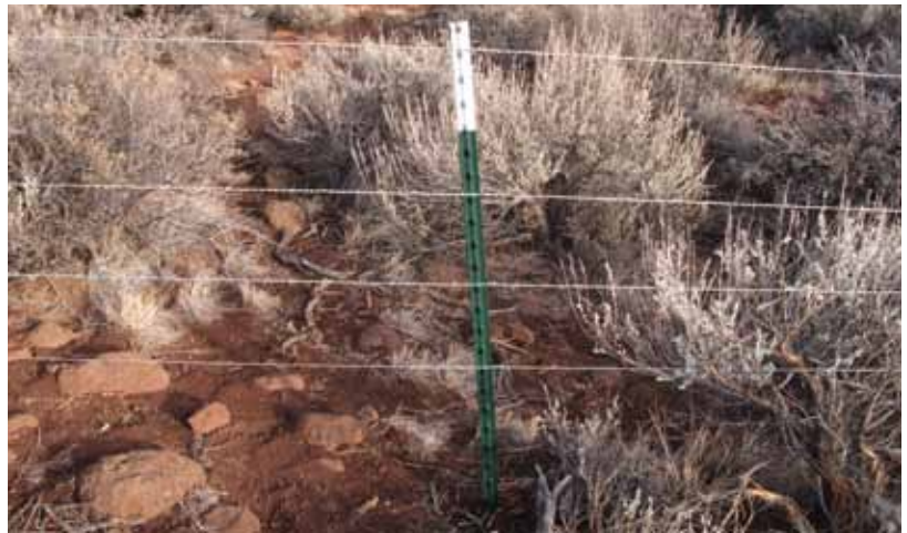
Note the smooth wire and large gap at the bottom of this fence so that pronghorn, sage grouse and other wildlife can get through to the other side safely.
