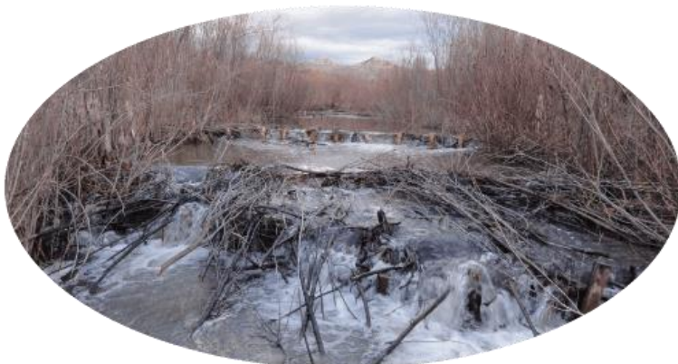
Left: A sequence of BDAs in a series, collectively forming a dam complex. Photo courtesy Anabranch Solutions
